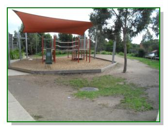
Gecko provided a solution by firstly excavating the area and setting some new ground levels. The existing surface was full of trip hazards and undulations. The storm water pit was also raised up and the high points were lowered creating a much more functional area.
