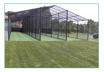
MSPRO45® Plush was used to form the run up area and the sturdy powdercoated nets were installed to form the protective net barriers. 10mm thick industrial rubber curtains were then hung to provide ball protection and reduce leaf and debris build up in the net area.
