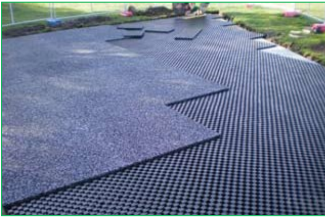
20mm Shockpads laid over Drainage-Cells
