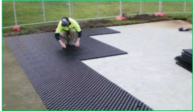
Installation of 30mm Drainage- Cell
