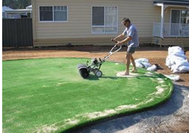
Installation in Progress
