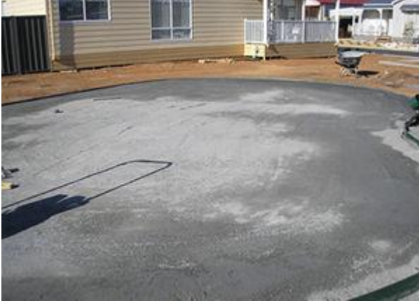
Laying the Base
